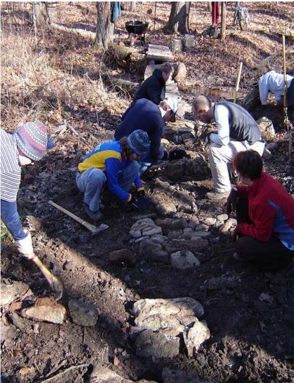
(e) Filling in the spaces with smaller rocks
