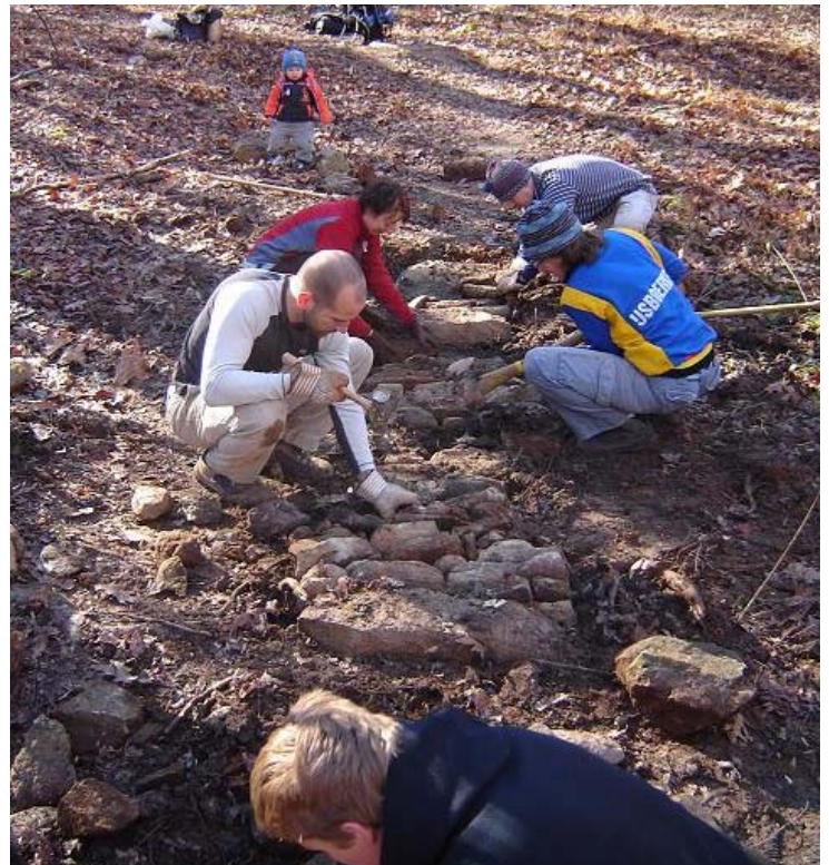
(e) Filling in the spaces with smaller rocks
