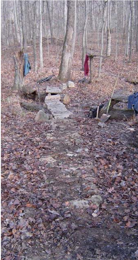
(f) The finished armored section
